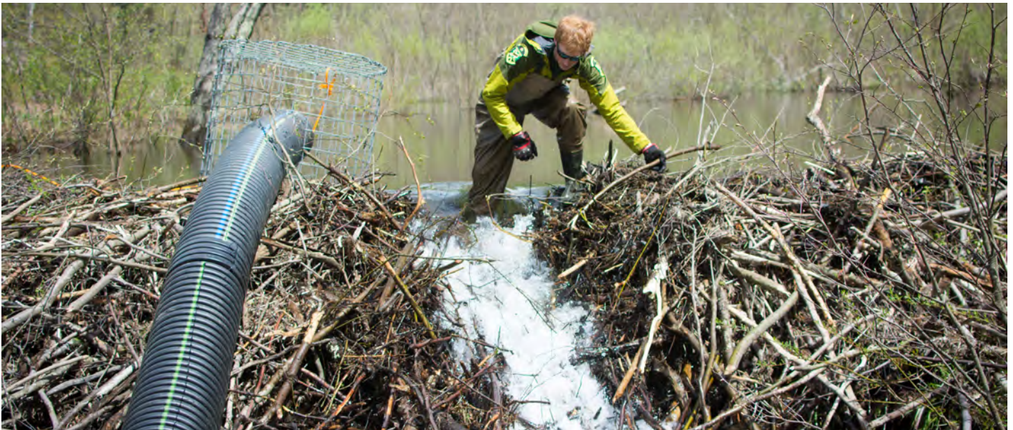
Wildlife Specialist Tyler Brown prepares a "beaver baffle," a device that allows water to pass through a dam without breaching it and destroying wetland. Baffles are one technique that Vermont Fish & Wildlife staff recommend to minimize beaver damage. Photo: Vermont Fish and Wildlife Department
