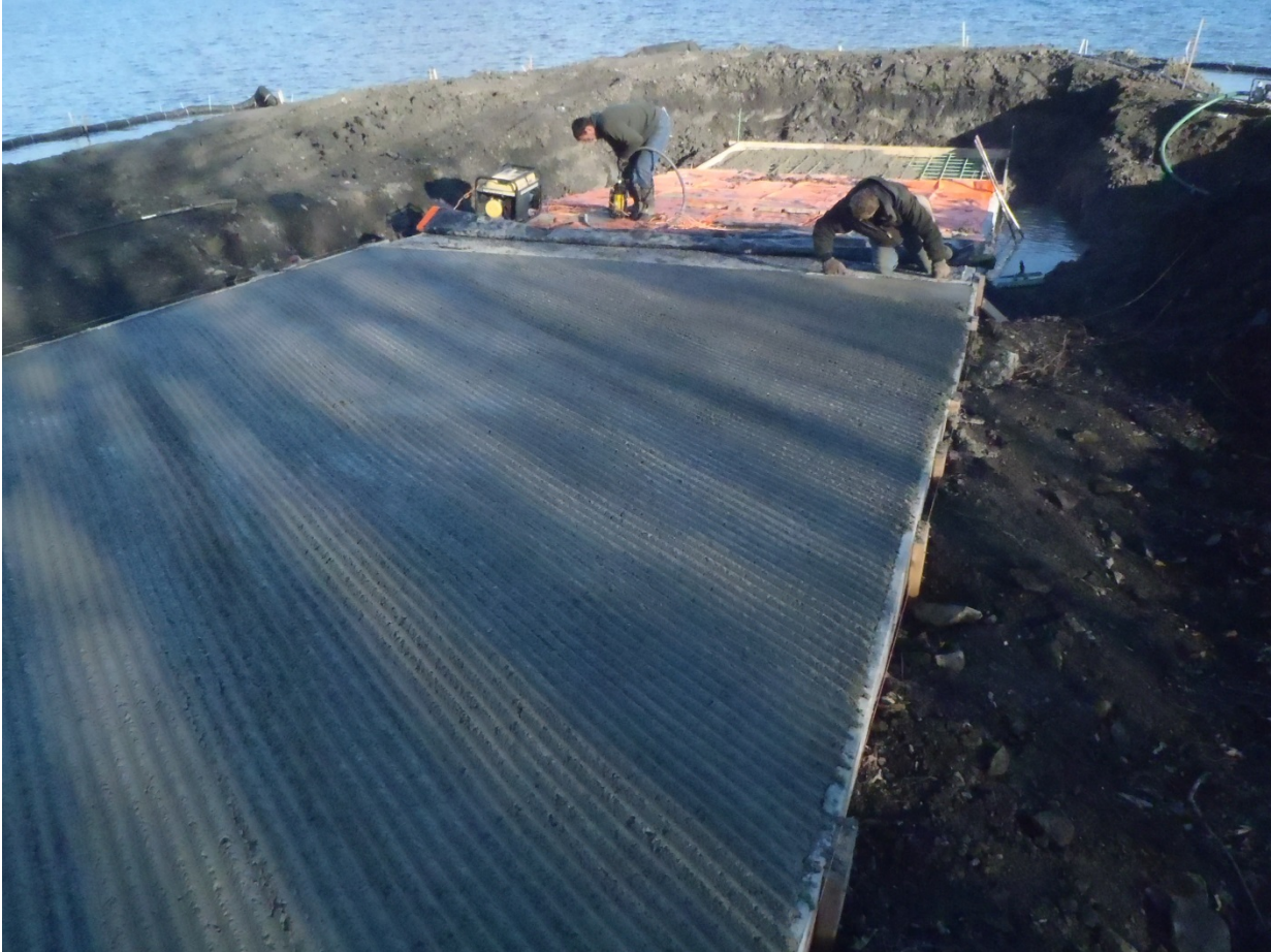
Figure 3. Pouring the concrete at the Dillenbeck Bay Fishing Access Area in Alburgh, VT. The ramp was formed and poured December 2016 and the project was completed April 2017. This popular fishing access area used to have a very shallow gravel ramp, which made launching at this site after early July difficult to impossible. Now anglers, boaters, and waterfowl hunters can utilize the ramp into the fall.
