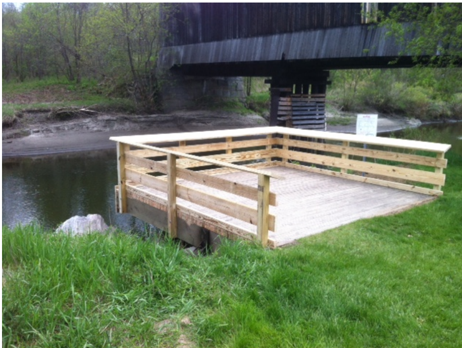
Figure 2. The rebuilt Fisher Bridge fishing platform, June 2016, Wolcott, VT.
