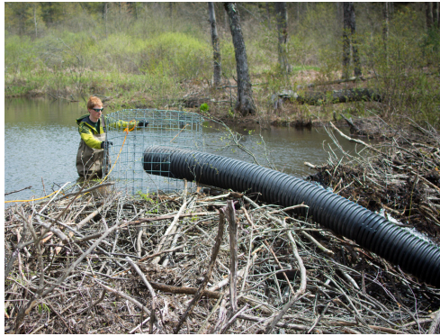
Above: beaver baffle Below: exclusion fence
