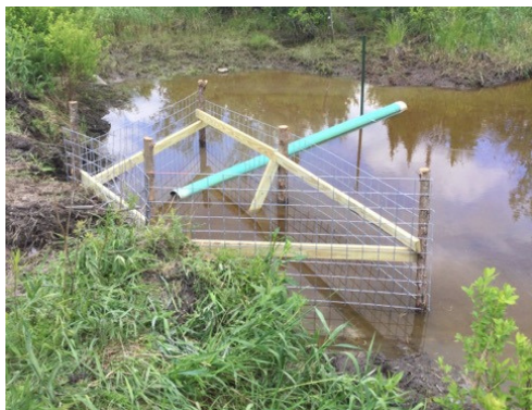
Above: beaver baffle Below: exclusion fence
